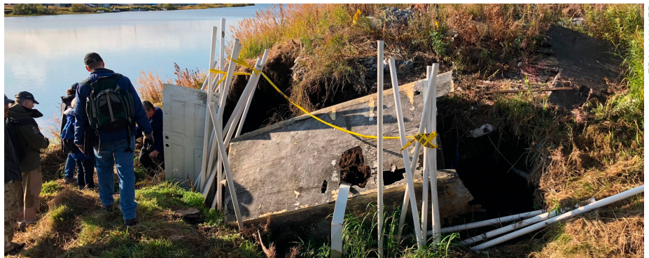
Building collapse due to permafrost thaw in Selwak, Alaska.
