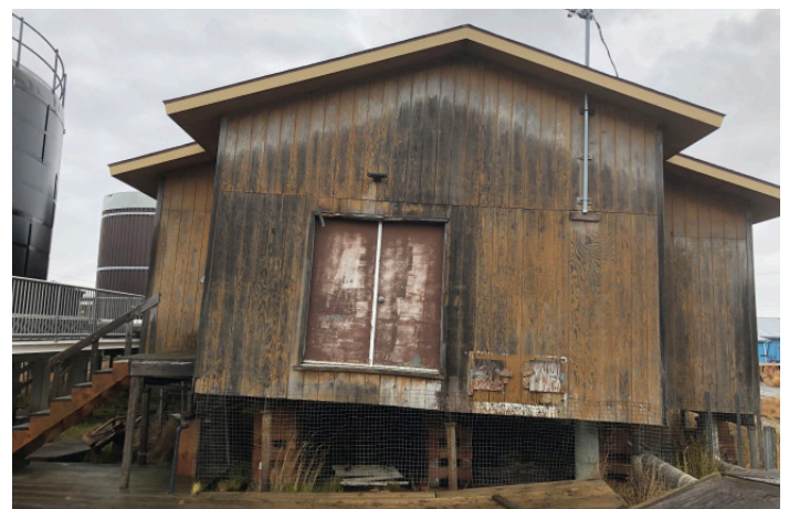
Foundation failure caused Nunapicuaq’s washeteria to temporarily close in 2022, leaving the village without running water for cleaning dishes, flushing toilets, and laundry. Photo: Susan Natali/Woodwell Climate Research Center.
